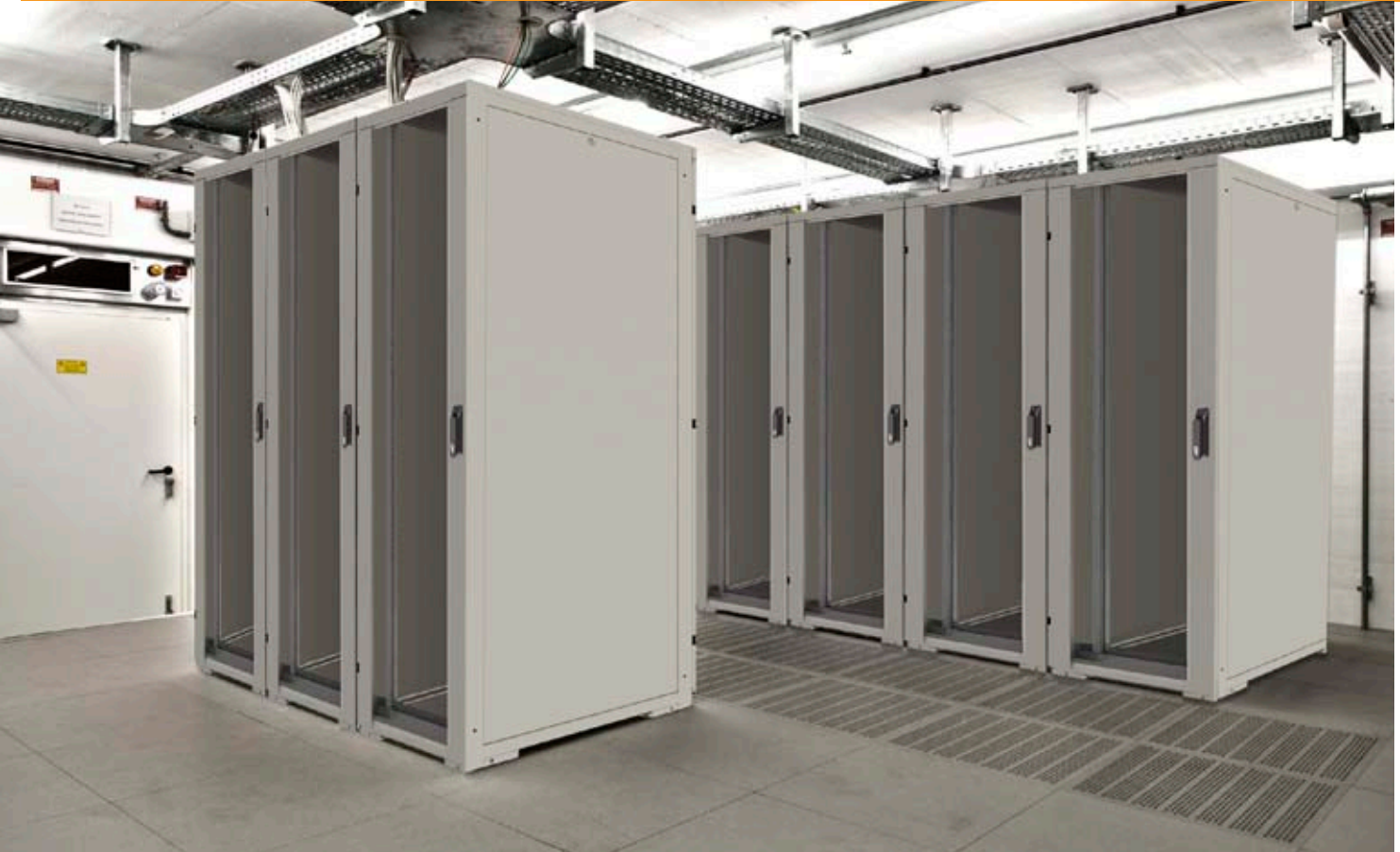
Standard racks being installed in a network room SME business
